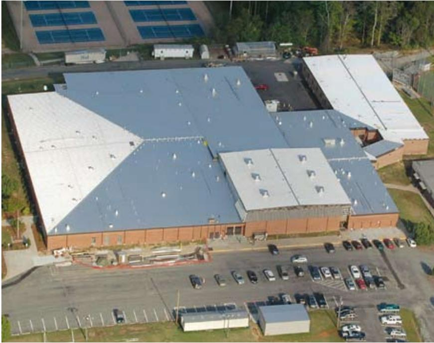
*Ledford High School (top) in Thomasville, N.C., with its new metal retrofit roof. At right is the leaky flat roof of Ledford before the installation of a metal retrofit roof.*
