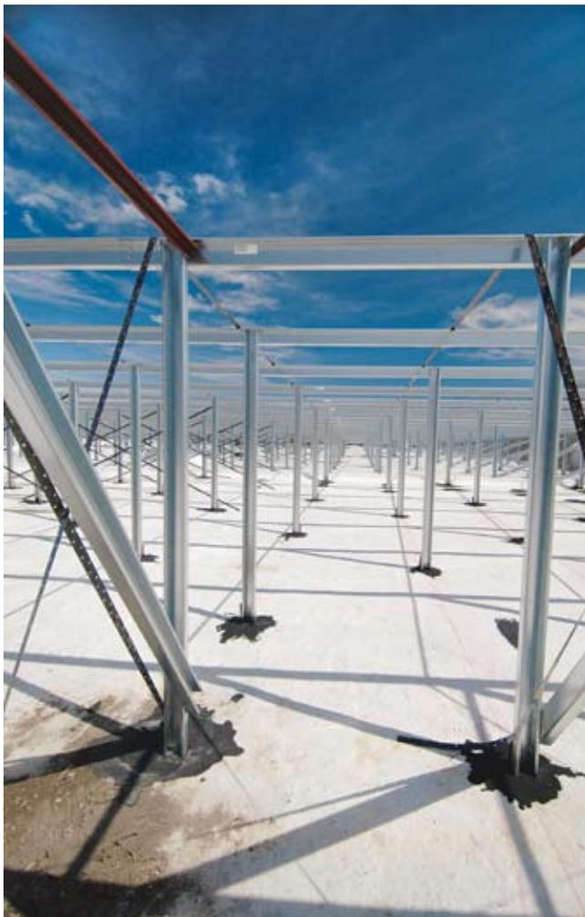
Subframing was attached to the flat roof of Ledford High School in preparation for a metal retrofit roof.
