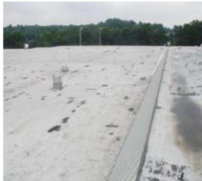
a metal roof panel was used for the weathering surface, water is allowed to flow freely to the building perimeter instead of ponding on the roof membrane. This fact, positive drainage, is the simple but most potent characteristic of a metal retrofit roof system that provides the greatest changes in the roof component of the building.
