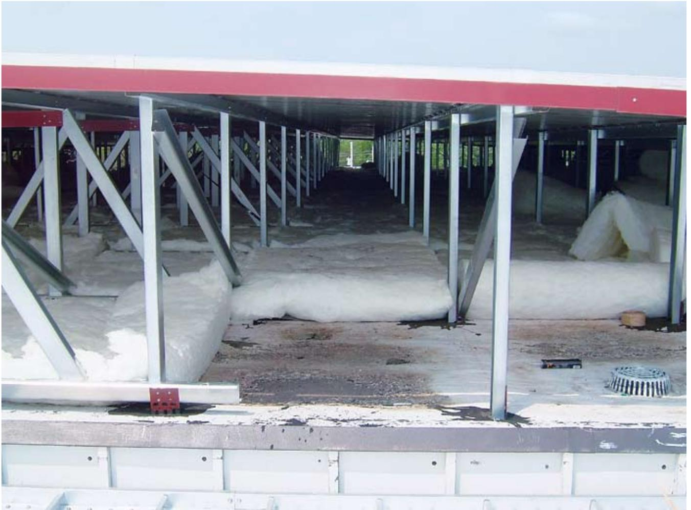
*This is the new roof cavity of Ledford High School in Thomasville, N.C., showing just-installed 6 inches of fiberglass insulation. This project is one of 15 in the Davidson County School District to be re-roofed with a retrofit metal roofing system. CHUCK HOWARD PHOTOS*
